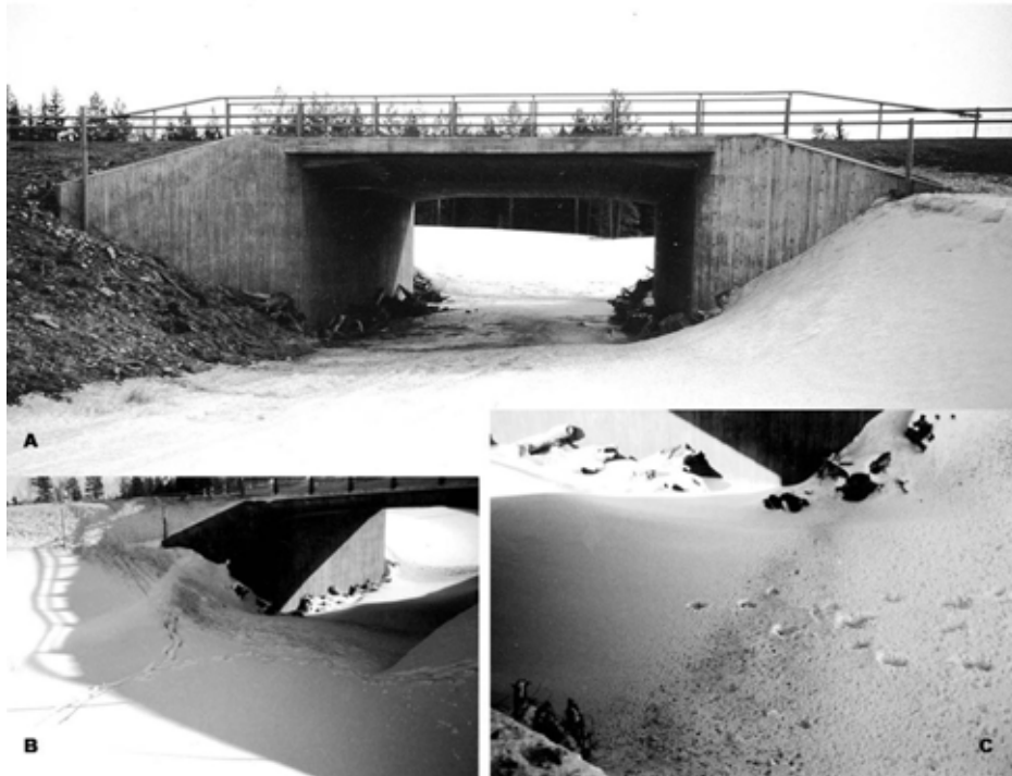
Figure 7.1 Moose snow tracks at the entrance of one of the moose underpasses constructed under highway E4 in the High Coast area in northern Sweden (A). Moose often avoided entering the underpass (B). Some individuals turned around exactly at the entrance (C). Snowtracks suggest that moose may have been scared away from the underpass, maybe by passing vehicles. (Photo: Erik Ringaby.)
