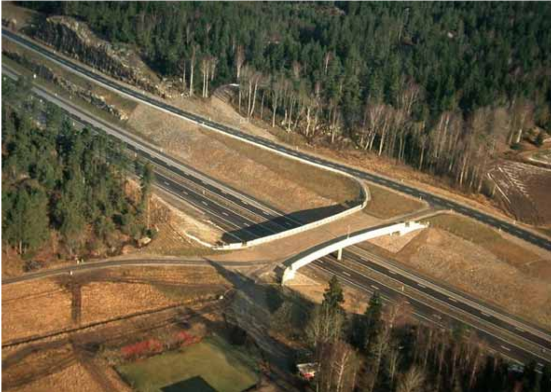
Figure 7.2 The first road overpass in Sweden adjusted for moose located at highway E6 near Uddevalla on the west coast. (Photo: Mattias Olsson.)
