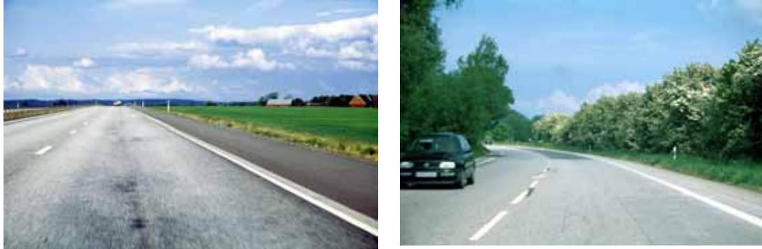
Figure 3.5 Verges can vary considerably between different landscapes and countries. Left: A motorway in southern Sweden consisting only of an open ditch. Toxins and salt from the road surface can easily spread onto the adjacent agricultural field. Right: A highway in Germany. Densely planted shrubs and trees along roads provide potential nesting sites for birds and screen the road and its traffic from the surrounding landscape. (Photos by A. Seiler.)
